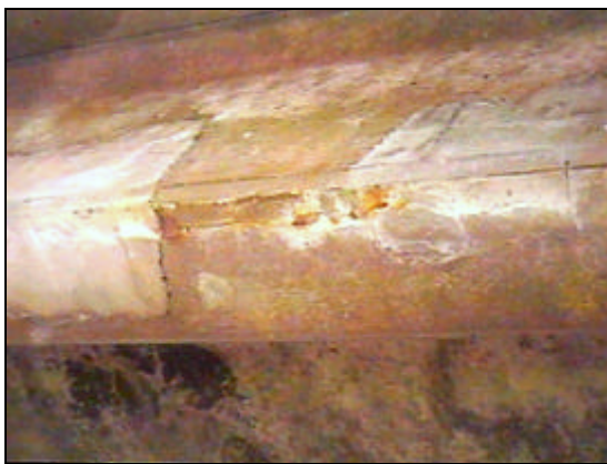
Previously repaired beam spalling.
