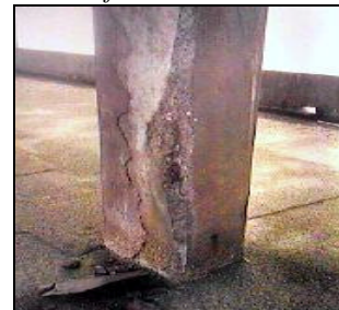
1984 repaired column, spalling in 1997.
